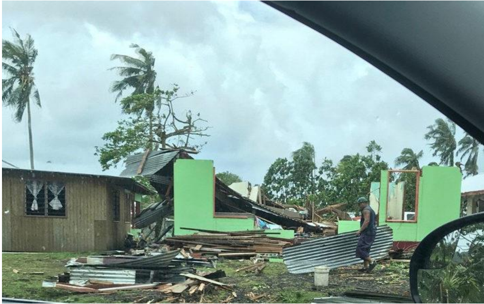
Figure 1-1. Damage from Cyclone Gita in American Samoa (Source: Radio New Zealand, 2018)
